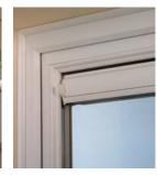
Trickle ventilators and night vent locking systems are the easier methods for providing ventilation when replacing windows. Where security is an issue or draughts will be a problem night vent locking systems are not recommended.
