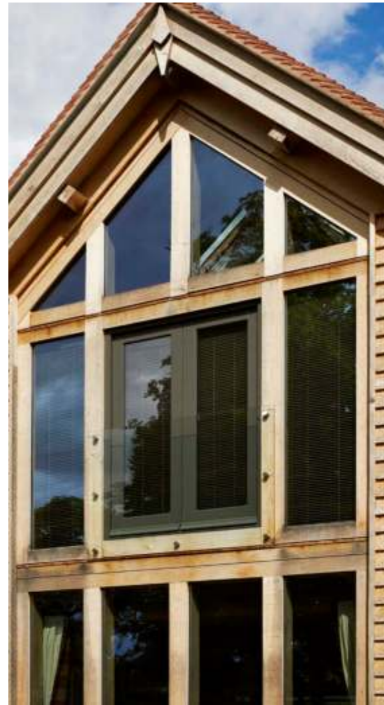
Flush casement windows painted in off white (RAL9010) and graphite black (RAL9011)
